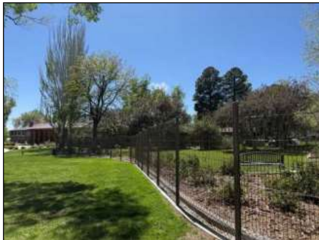
Construction Complete April 2026, Fuller Lodge in Distance
